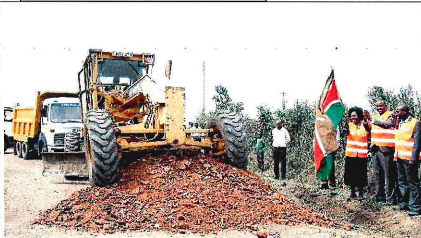
Kamongil-Kamosiro-Kaboson road, under construction
