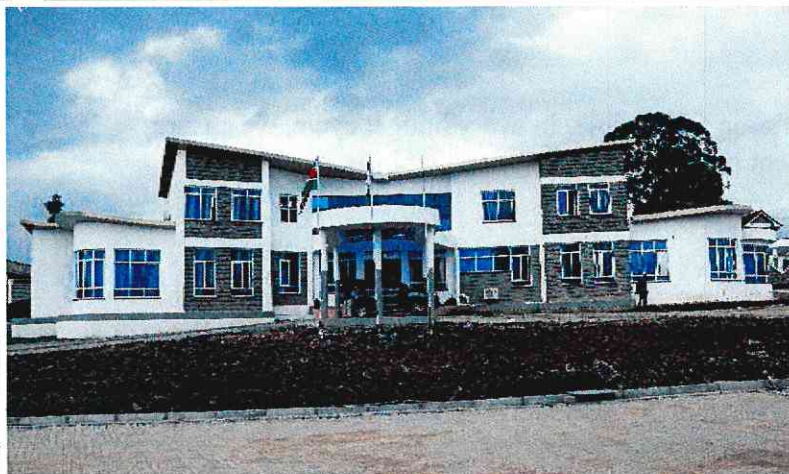
Completed Administration block
