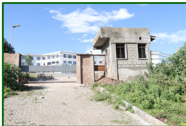
Main Gate and Gate house
