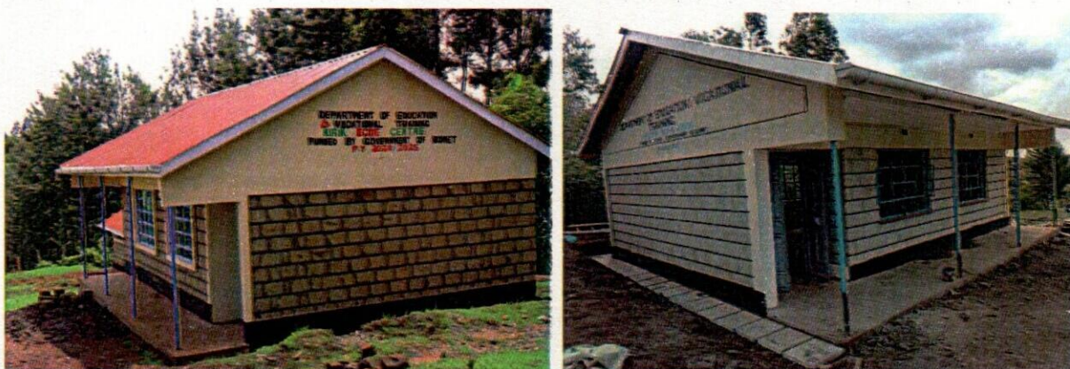
Fig. 1 Completed ECD classrooms
